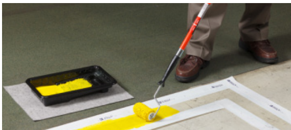
Paintstripe & floor marking area
