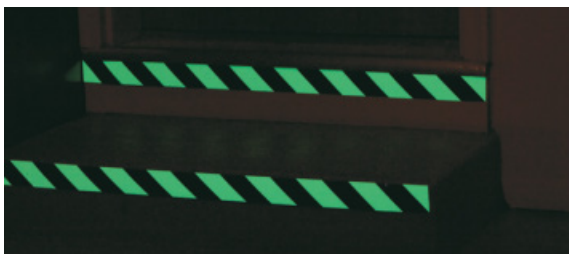
Photoluminescent area marking
