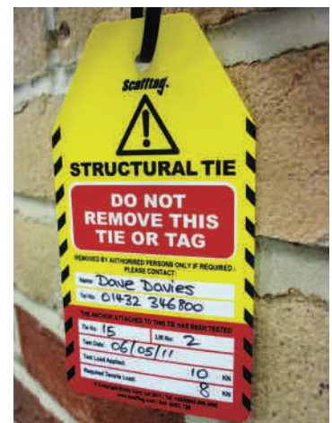
Legend: Do Not Remove Scaffold Tie
