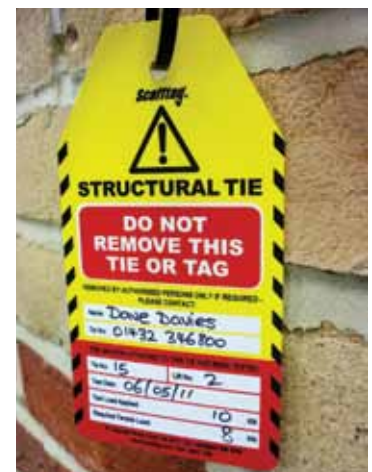
Legend: Do Not Remove Scaffold Tie
