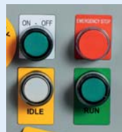
Control Panel Labelling
