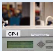
Control Panel and Electrical Panel Labels
