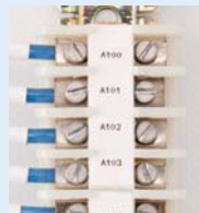
Terminal Block Marking
