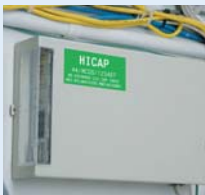
Control Panel Labelling
