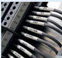
Wire & Cable Marking
